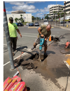
The Army is Power Washing and the Airforce is Power Drilling!
